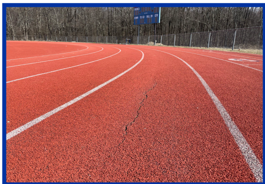
The track is used by our Modified and Varsity Track teams and is enjoyed by the community. Visible cracking is prevalent across many areas of the track.
